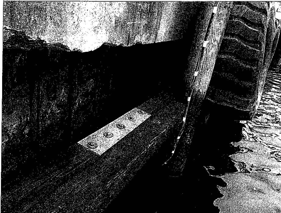
Photograph 3: Typical bulkhead/fender construction
