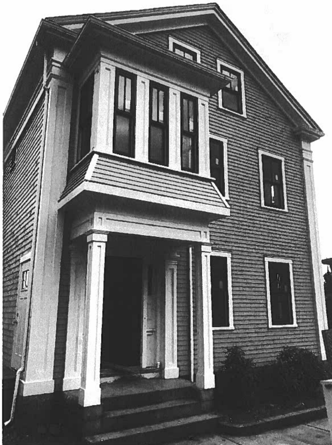
1060 Pleasant Street- West Elevation
