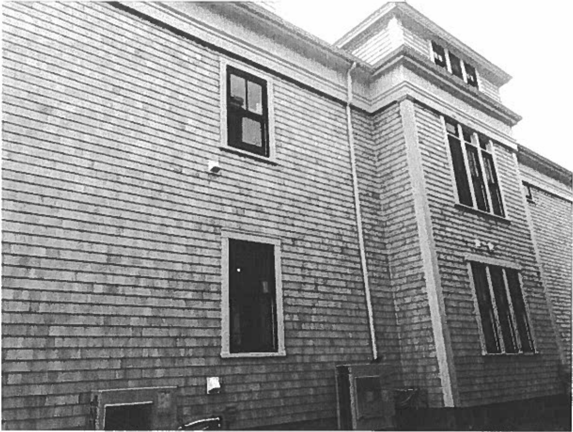
1060 Pleasant Street- Rear Ell North Elevation
