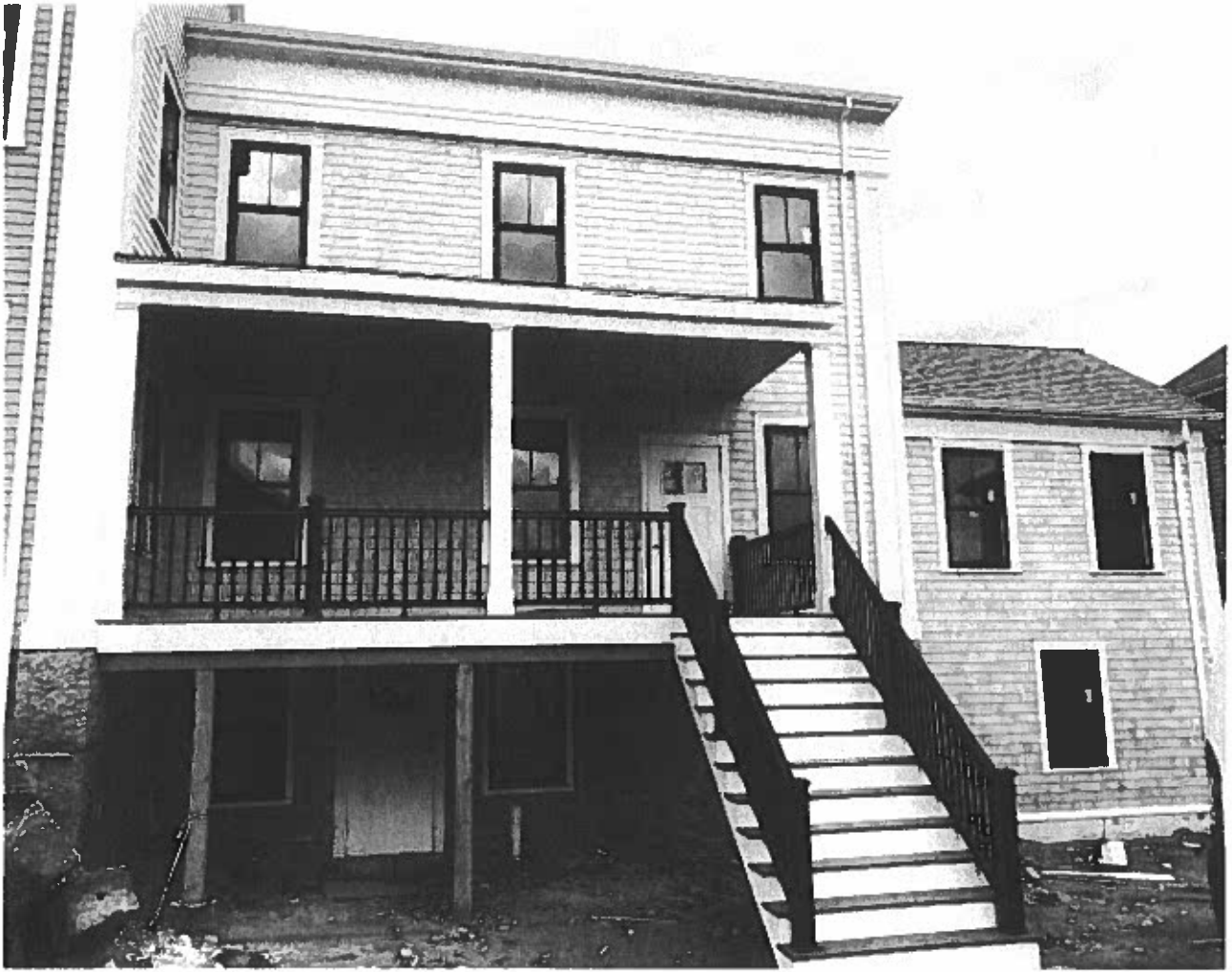
1060 Pleasant Street- Rear Ell South Elevation
