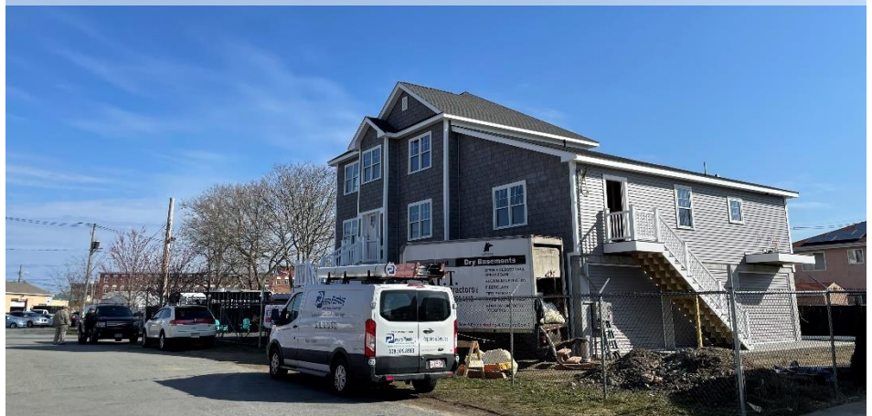
Lot 85 & 86 Residence under construction. Looking north-northeast on Osborn Street.
