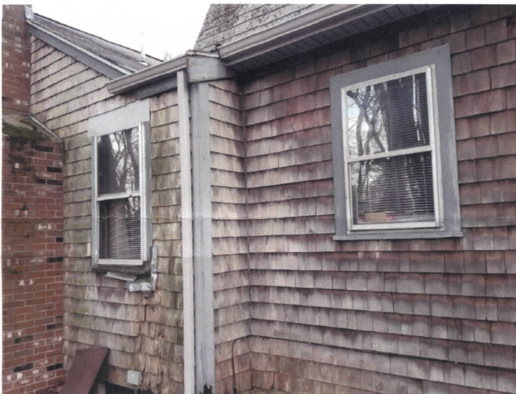
Example of deteriorated exterior envelope.
